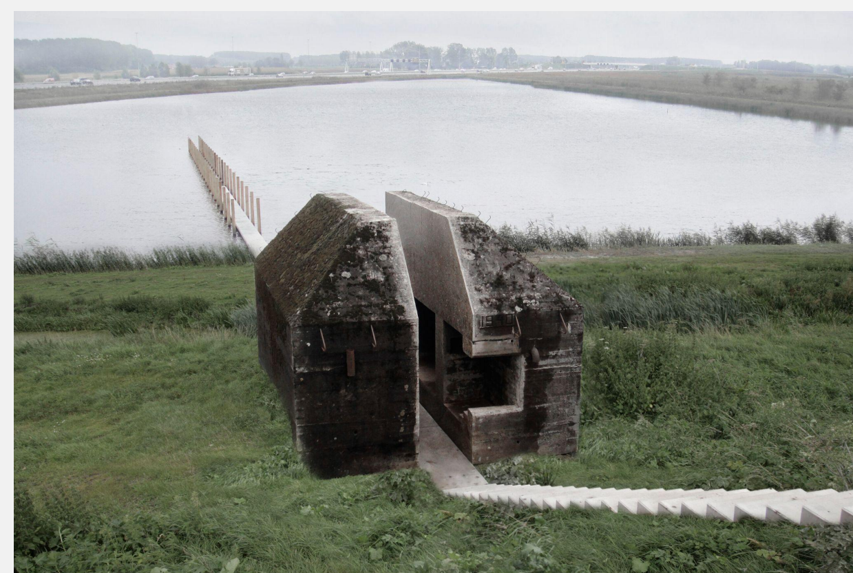
Bunker 599: Site Perspective
